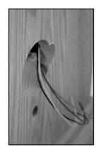
Pull wires from hinge side of door and out of 2-1/8" through hole.
